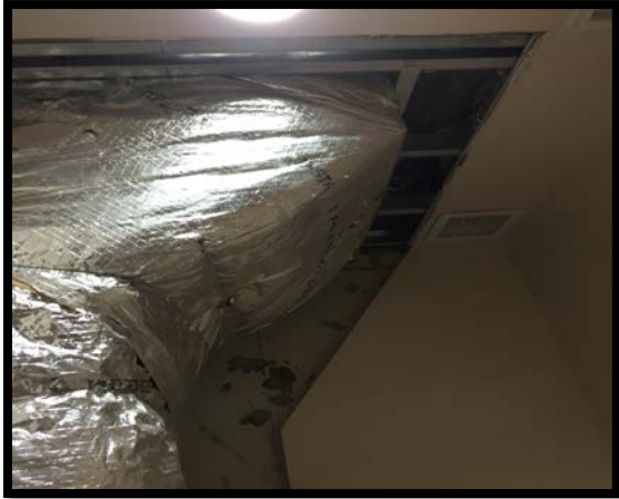
Level B AHU Duct Tie-in
