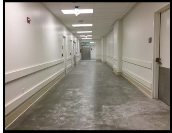
Level B Flooring and Base Installation
