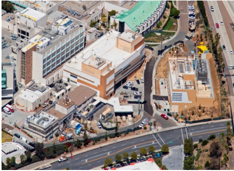
Aerial Photo of the new H&V and CEP
