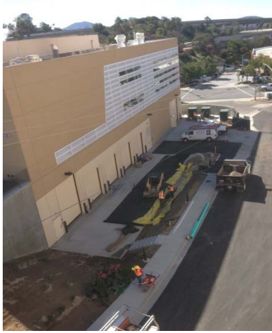
Newly Paved road between H&V and CEP
