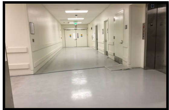
Level B Floor Oil Repair Work
