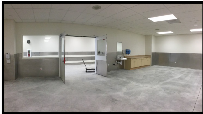
Level B Floor Prep Work
