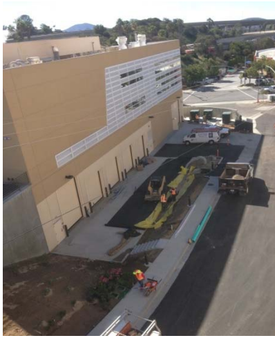
Newly Paved road between H&V and CEP
