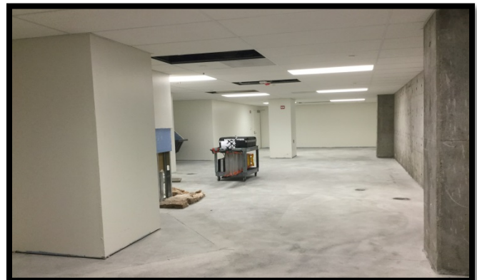
Level B P-tube Storage Room
