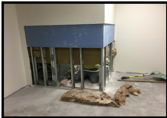
Level B Restroom Oil Repair Work
