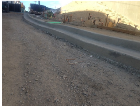
Curb and Gutter along ring road
