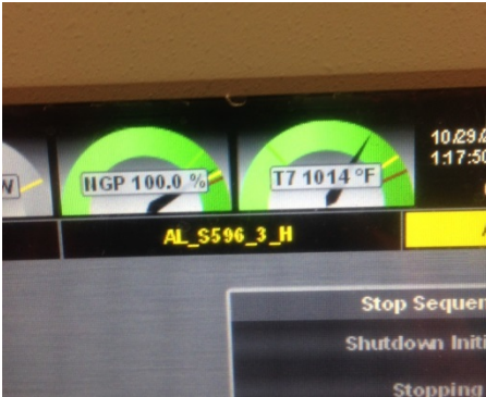
Turbine Control Showing it is running at 100%
