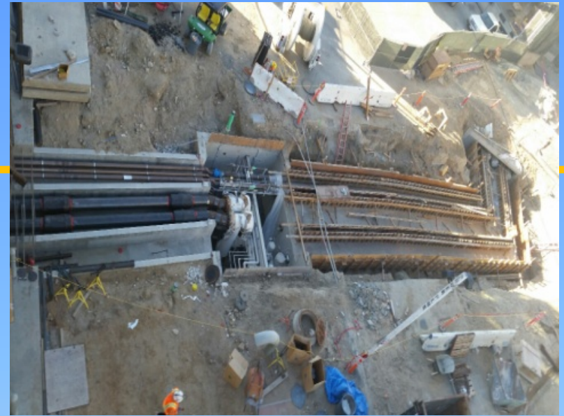
Utility Tunnel Connection
