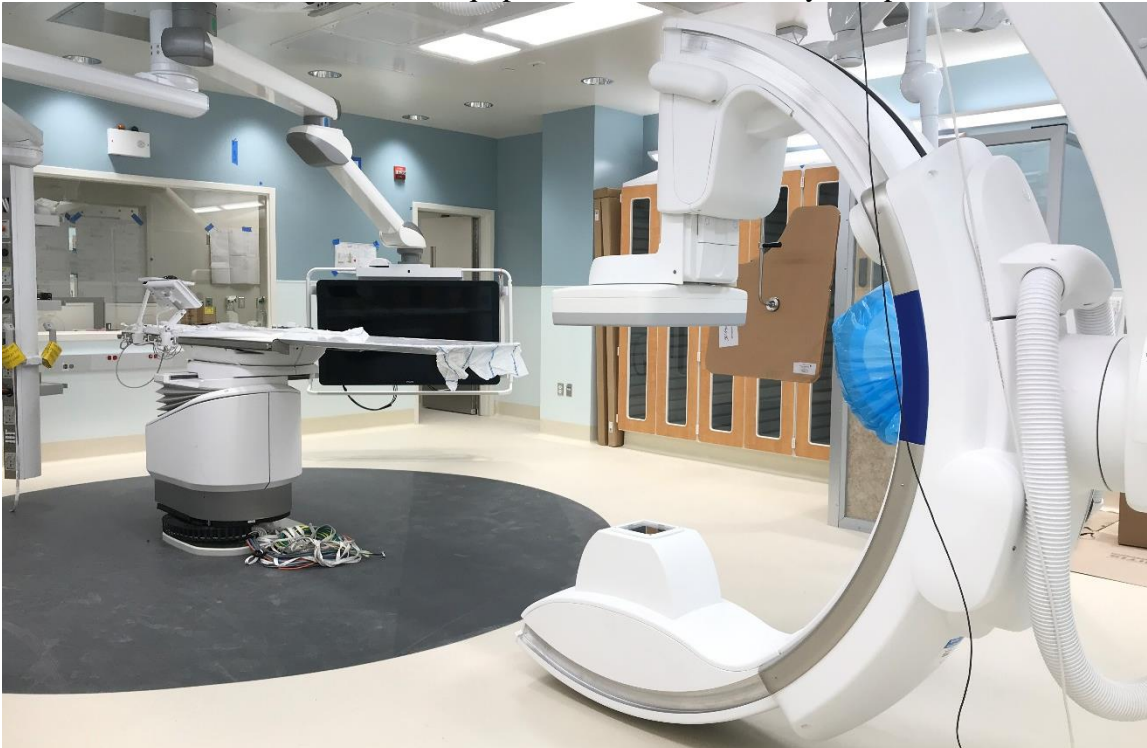
5-16-18: Cath Lab #1032: Medical equipment installation complete.
