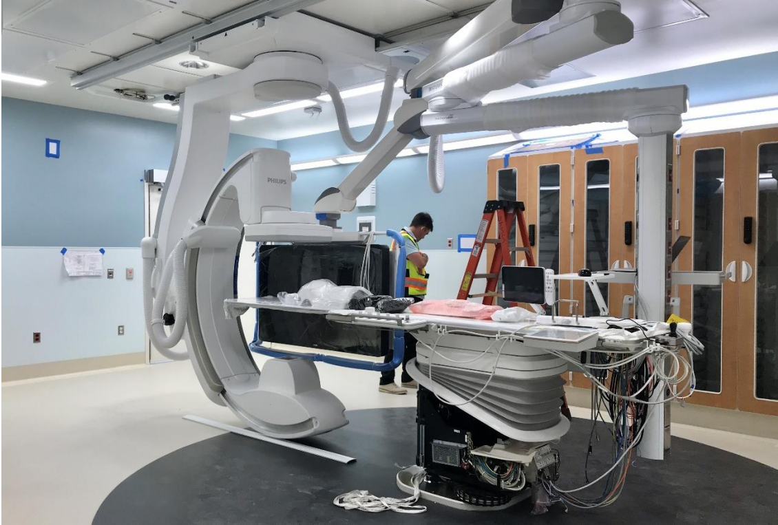
5-23-18: Cath Lab #1024 Medical equipment installation nearly complete.
