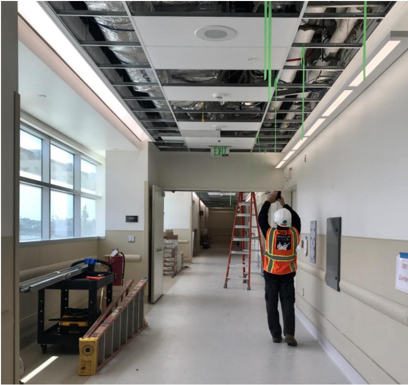
5-23-18: East Corridor: Getting ready to install the last ceiling tiles.
