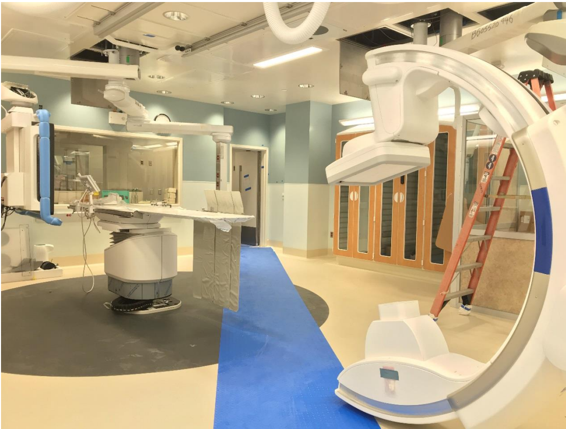
4-24-18: Cath Lab #1023 Medical equipment installation nearly complete.
