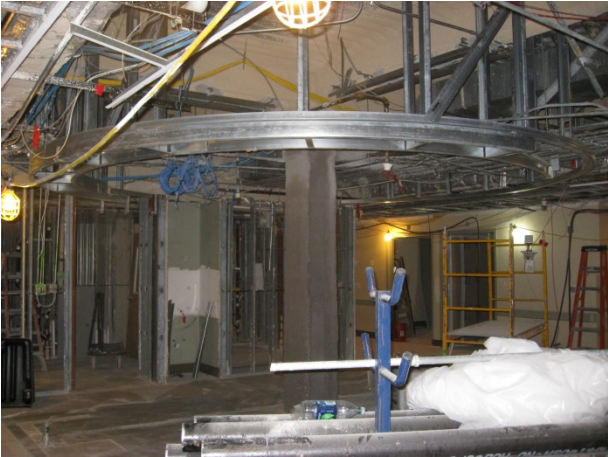
Photo #1: Central Nurse Station Demo and Ceiling Soffit Framing
