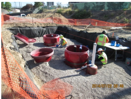
Underground Fuel Tank Installation
