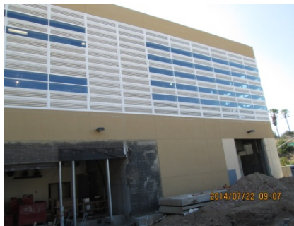
Curtain wall and Louver
