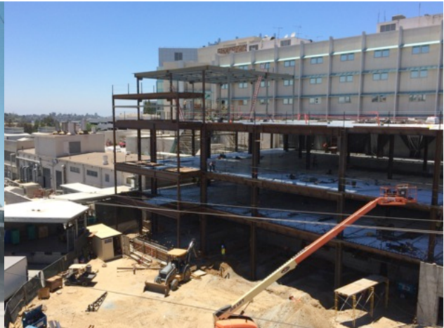
Completed structural steel frame and metal deck.
