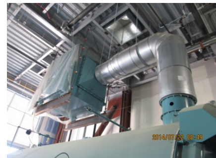
Boiler and Flue Installation
