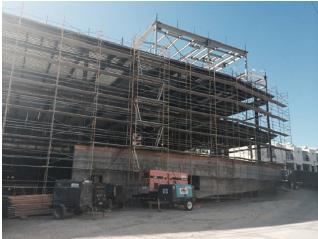
Scaffolding is in place for exterior skin installation.
