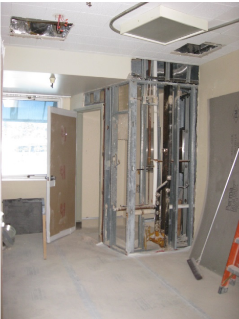
Photos #4 & #5: Single Patient Room Demolition
