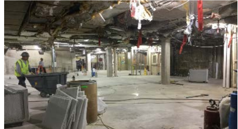
Level 1 Wall, Flooring, Ceiling Demo
