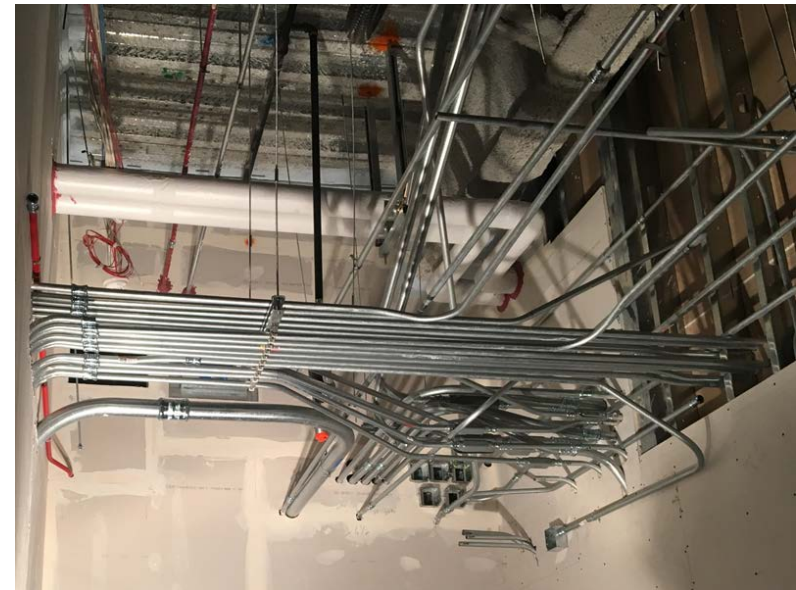
Control Rooms: Overhead Electrical Nearing Completion
