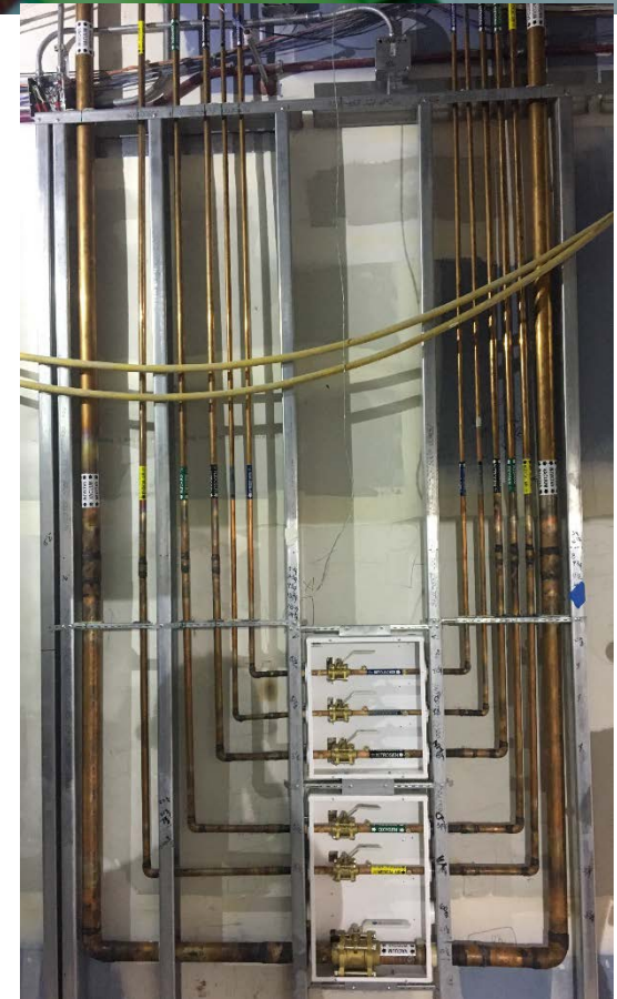
Medical Gas Zone Valves, Complete
