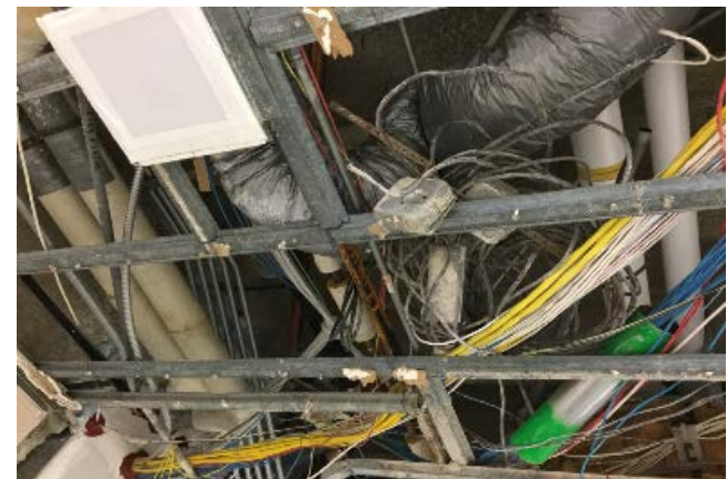
Level 1 Ceiling Existing Conditions
