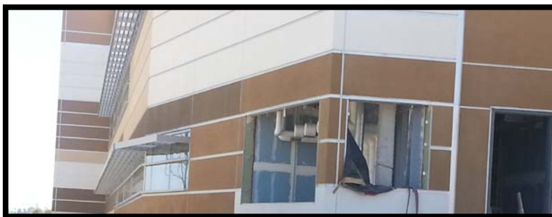
Exterior Louver Repairs
