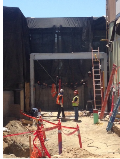
Trellis Structural Steel Work
