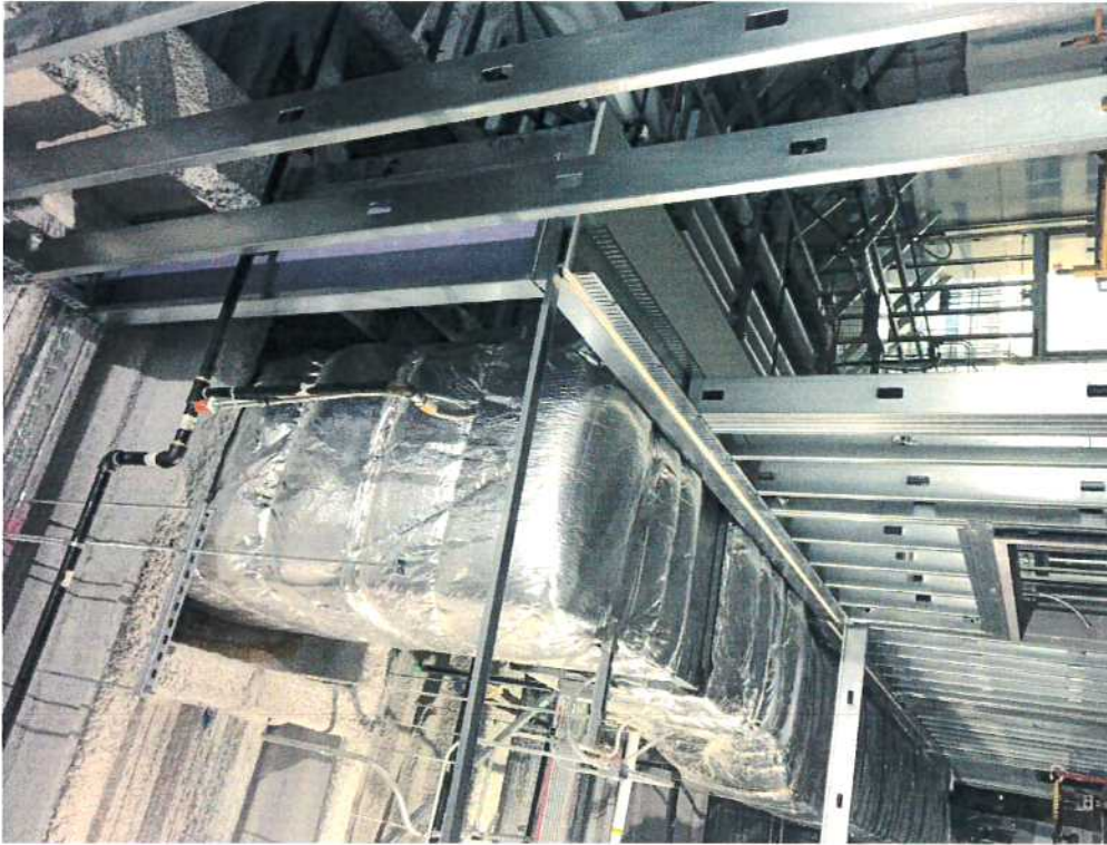
7-19-2017: Furring around mechanical ductwork conflicts in walls.
