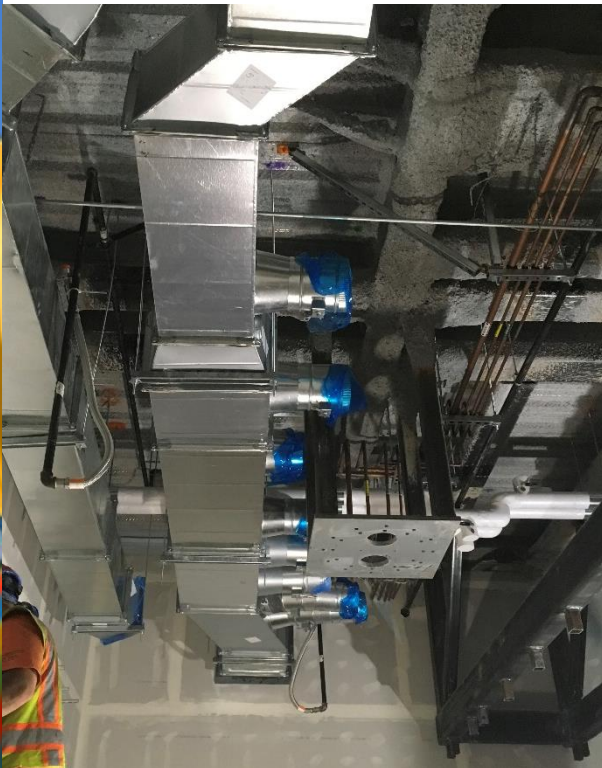
Cath Lab #1025: Mechanical ductwork installation in progress
