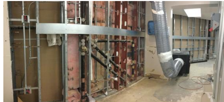
Level B Sterile Processing Reverse Osmosis/Deionized System Installation
