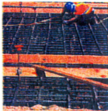
Reinforcing steel is set and ready for concrete
