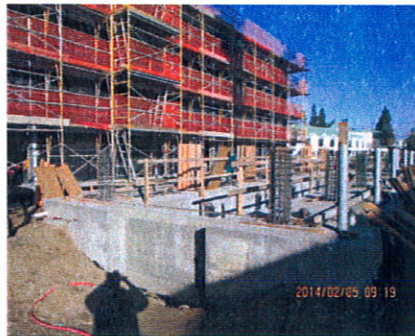
Cooling Tower Foundation & East Elevation
