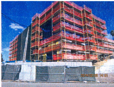
South and East Elevations
