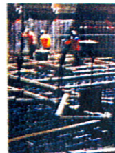
Reinforcing steel is set and ready for concrete
