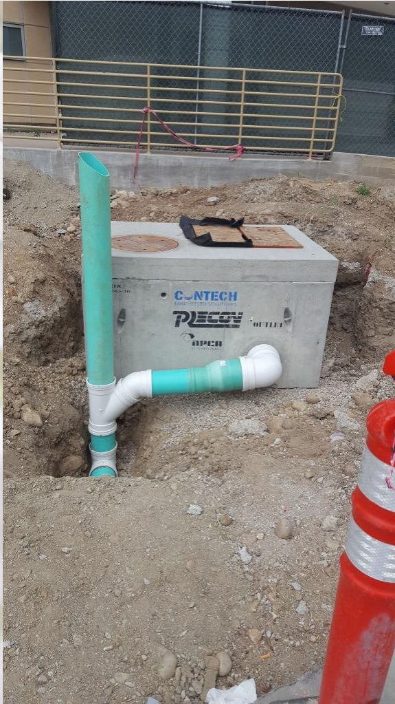
Storm Drain Inlet at Steam Line Trench Installed
