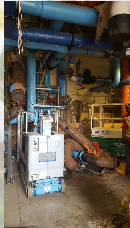
Demo In Existing Plant
