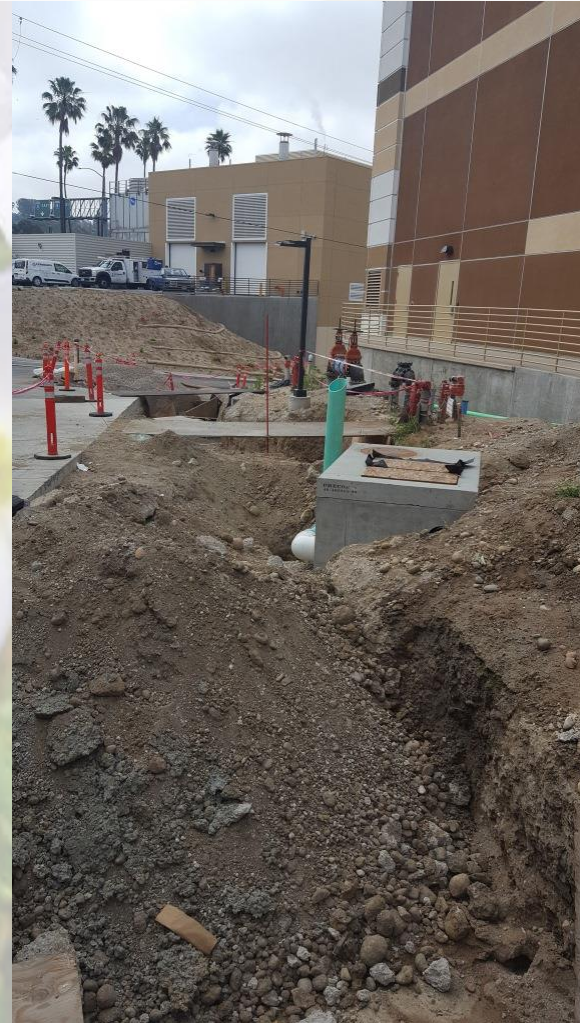
Storm Drain Inlet at Steam Line Trench Installed
