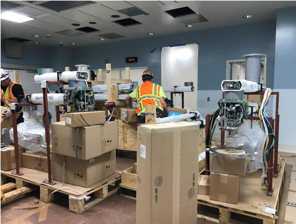
2-20-18: OR #1029 (Hybrid OR) Overhead Medical Equipment delivered
