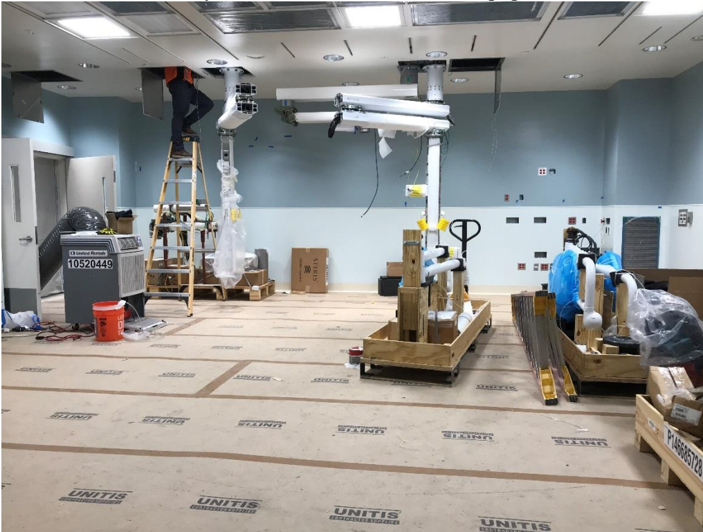
2-15-18: OR #1030 (Hybrid OR) Overhead Medical Equipment installation underway
