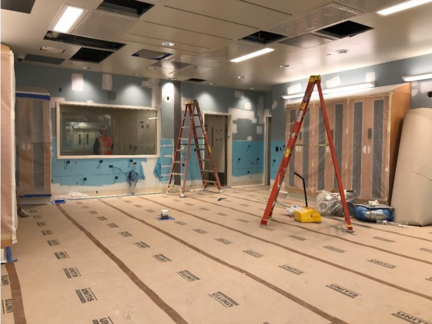
2-15-18: Cath Lab #1024: Wall protection complete, cabinets installed; finish flooring complete
