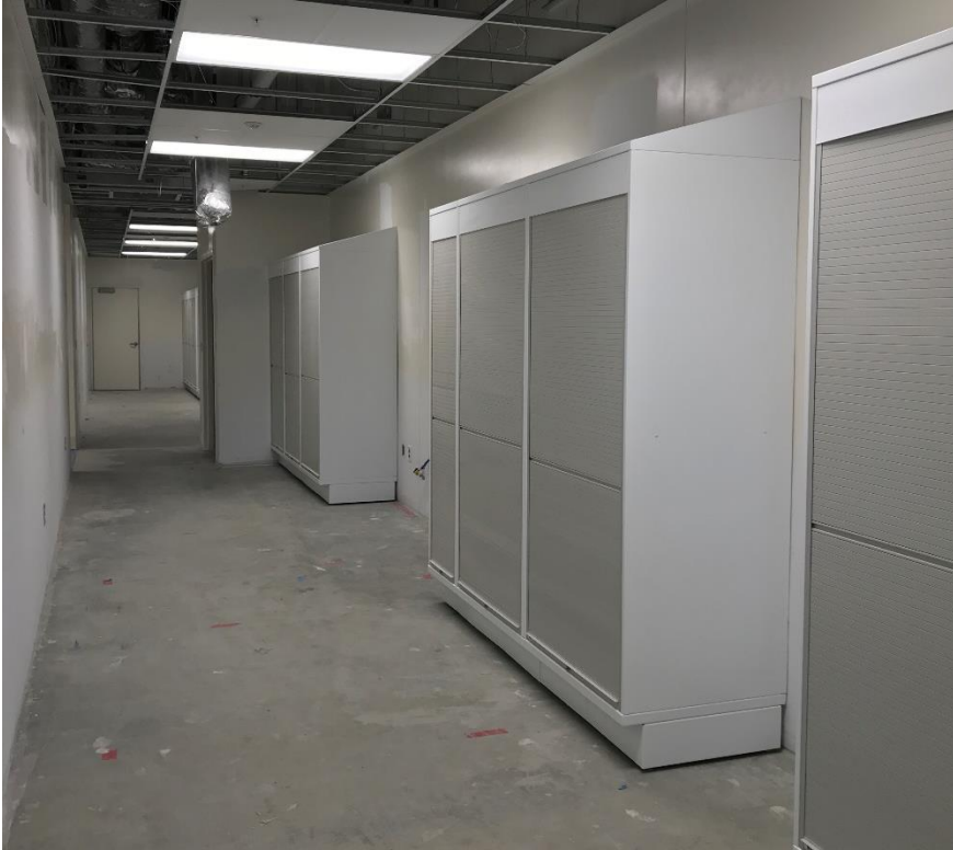
2-20-18: Cath Work Storage Area: Cabinets delivered, installed
