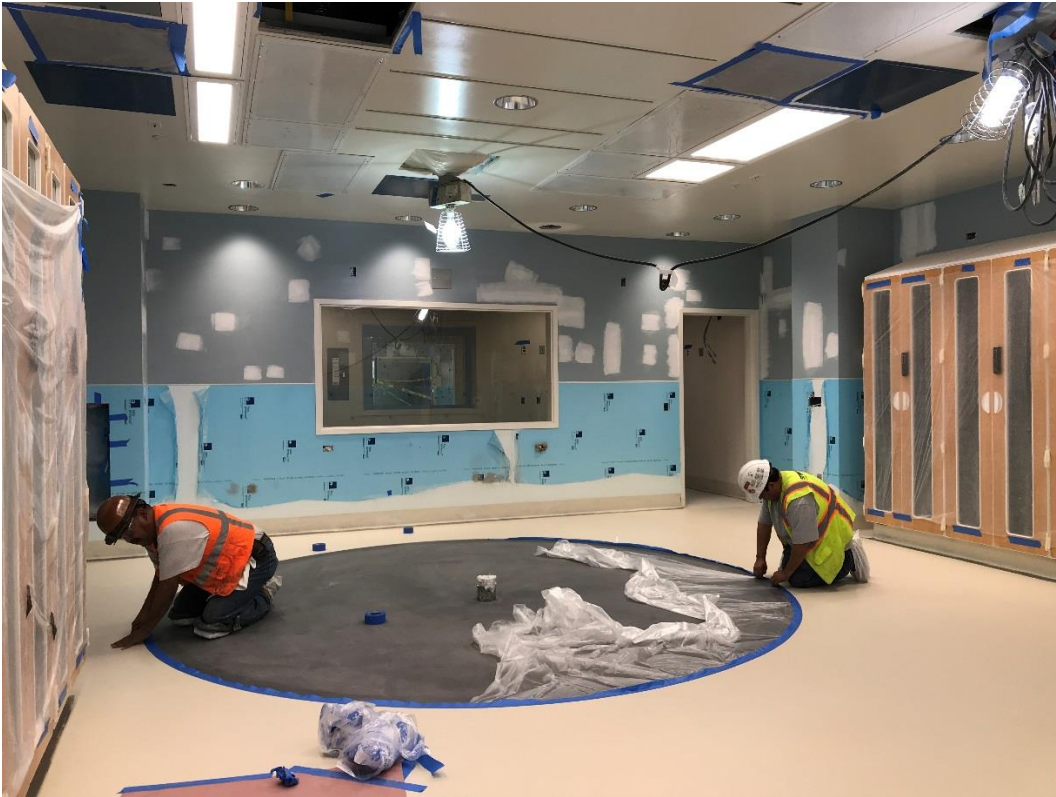
2-6-18: Cath Lab #1032: Finish flooring completed on 2-13.
