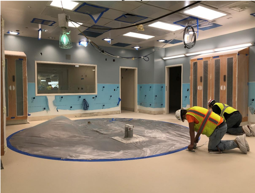
2-6-18: Cath Lab #1033: Finish flooring completed on 2-13.
