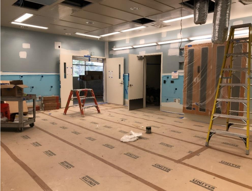
2-15-18: Cath Lab #1023: Wall protection complete, cabinets installed; finish flooring complete
