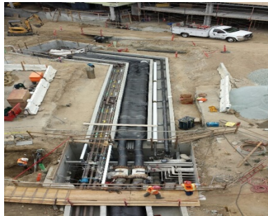
Utility Tunnel being fitted out with piping
