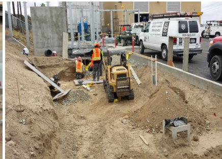
North site trash enclosure bio-swale
