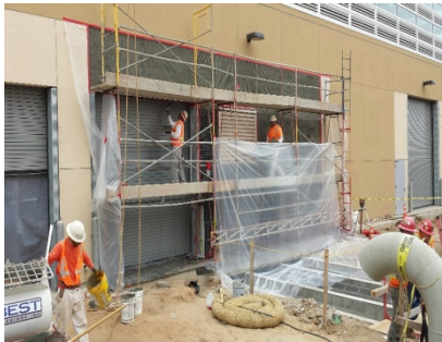
Stucco above utility tunnel
