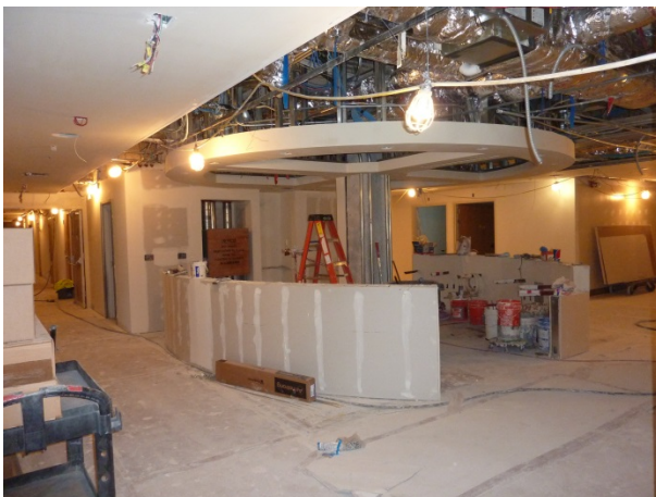
Central Nurses' Station, drywall installation
