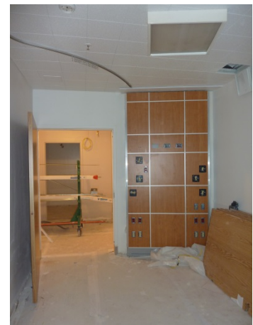
New Headwall in Patient Room
