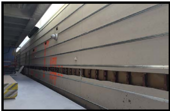
Level 1 Expansion Joint on East Tower
