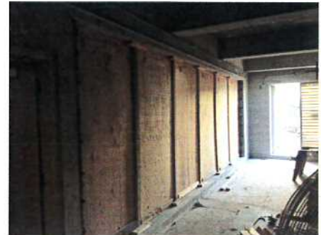
HVSB wall has been removed.
