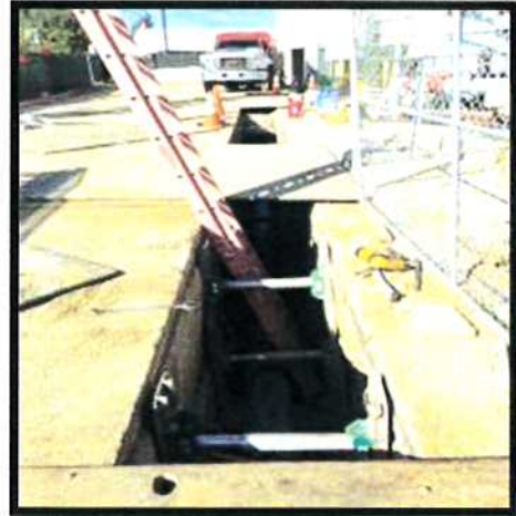
Helix Water Line Install
