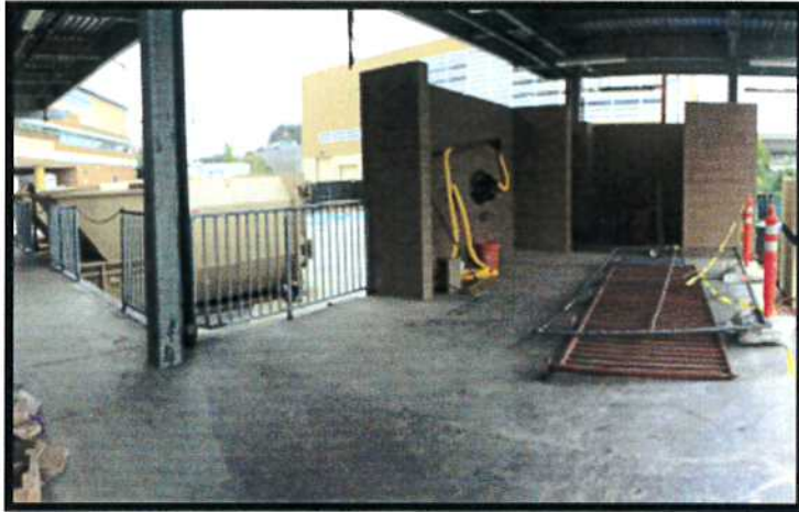
South Loading Dock Install
