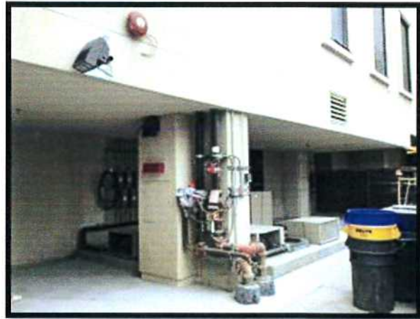
H&V North IAHU1 Ceiling Soffit Work
