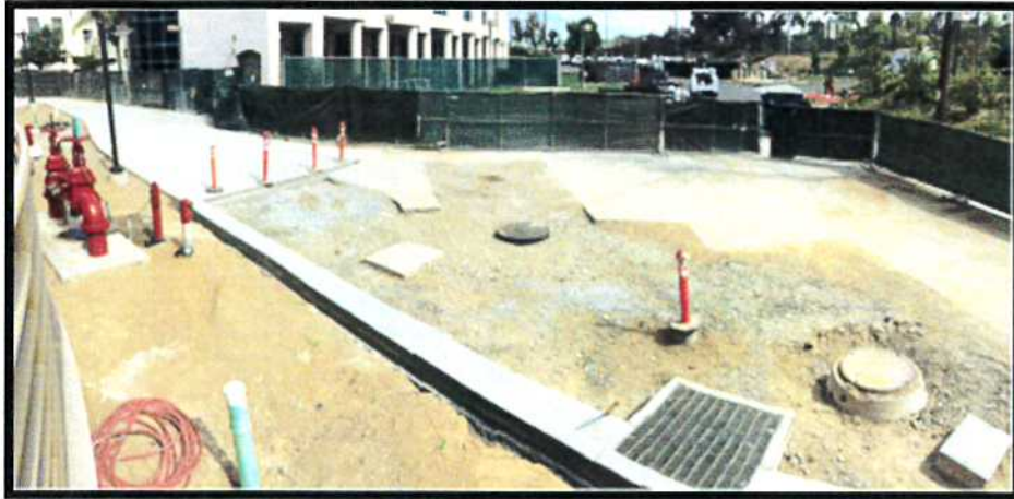
North Hardscape and Road Work
