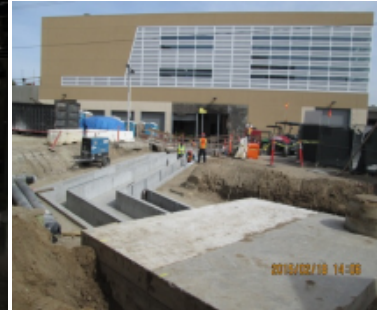
Utility Tunnel and West Façade
