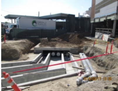
Site Work at H&V Vault
