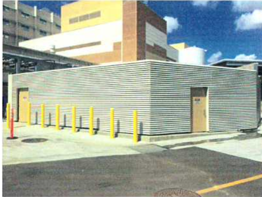
Bulk O 2 Enclosure Existing
