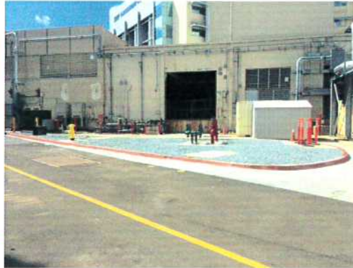
Old Soft Water System Location
