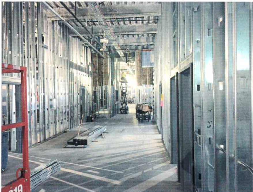
Central sterile corridor, looking north.
