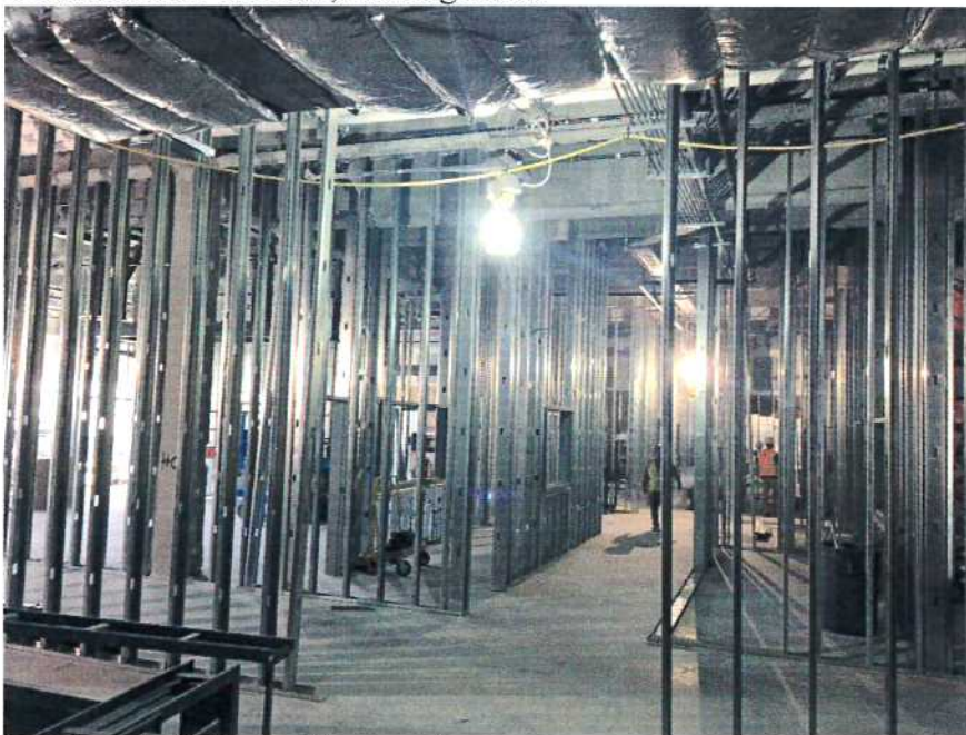
North end of site, looking south.
