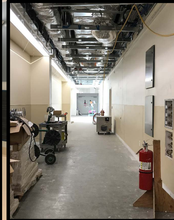
South Corridor: Lights installed; bracing ready for T-Bar grid supports
