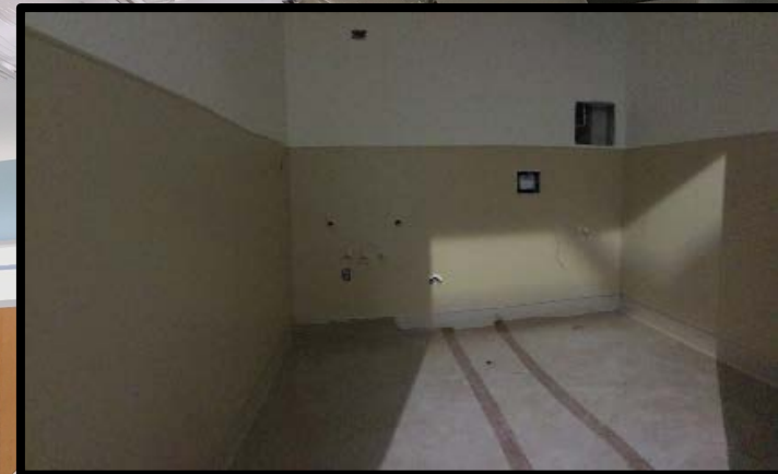
Install Floor & Wall Protection
