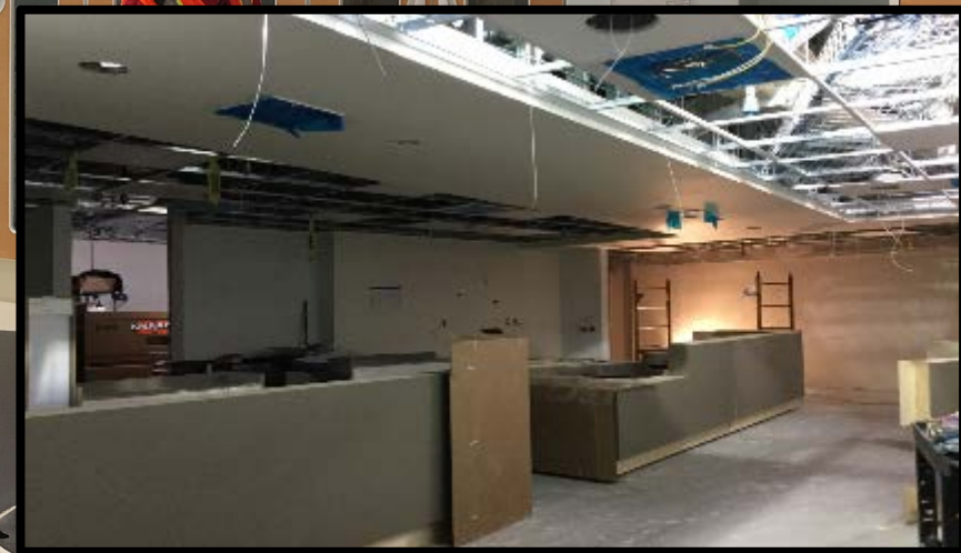
Central Nurse Control Station Casework Install
